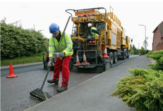
Machine applied Microsurfacing
