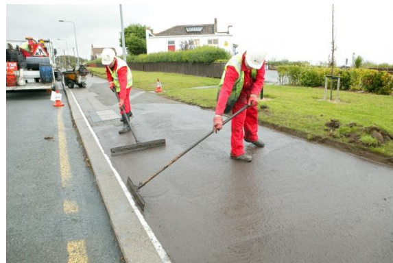
Hand applied Slurry surfacing
