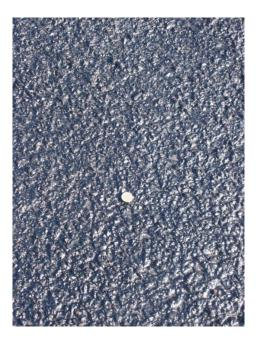
Over a period of time, the action of traffic on the Fortseal System exposes the microtexture of the aggregate restoring it to the original colour and texture, with the Fortseal remaining in the macrotexture of the surface acting as a Preservative and retarding the weathering process.
