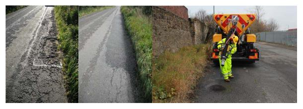
Velocity road repairs are a fast and efficient way to improve the network as the process does not cause any further damage to the road base and the simple but effective solution cleans, seals and repairs road damage extending the life of the carriageway and preventing the main cause of carriageway failure – water from penetrating damaged carriageway.
