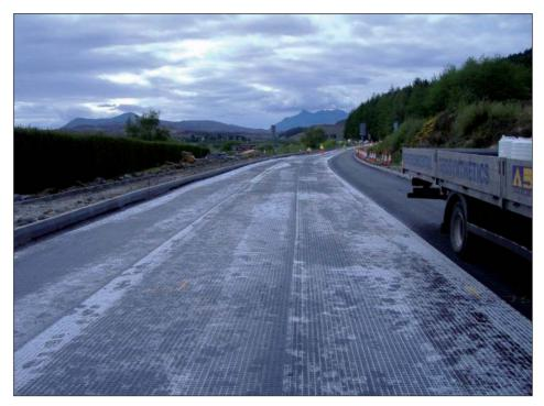
Rotaflex is installed using a K1-70 emulsion which bleeds through an integral polyester geotextile to ensure an excellent bond during installation with no movement during the paving process. The use of K1-70 combined with the open aperture structure of Rotaflex also ensures an excellent long term bond between all bound layers maximising pavement design life.
