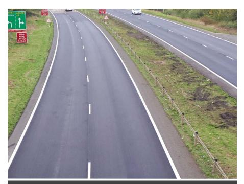
RHiNOPHALT® was spray applied to 38,500m<sup>2</sup> over several night shifts in October 2019, with 24,000m<sup>2</sup> treated in a single shift.
