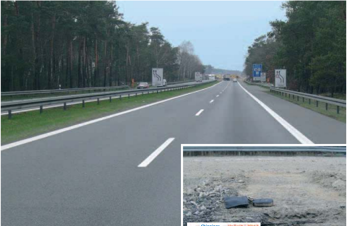
Condition of the German Highway 13 carriageway surface in 2005
