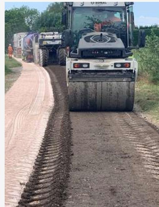
Where end of life roads are being surfaced they could be enhanced and made more resilient by the use of **geosynthetics and steel meshes** between replacement asphalt layers (typically below the surface or binder course), which will protect against future reflective cracking.
