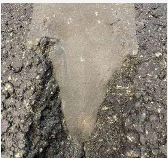
There's even been a departure from repairing failing joints (and cracks), which are often left until its fully fretted out and repaired as a safety defect and patched (introducing four joints, which could be susceptible to failure). **Crack and joint repairs** are simple and cost effective
