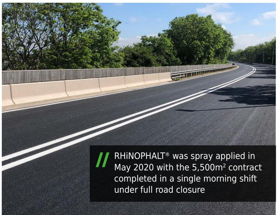
// RHINOPHALT® was spray applied in May 2020 with the 5,500m<sup>2</sup> contract completed in a single morning shift under full road closure
