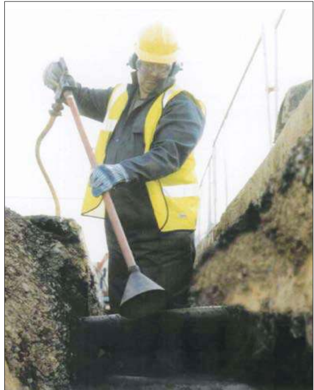
Figure 7 Using an air digging tool
