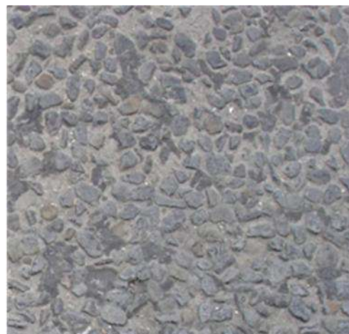
2011 – Showing repair in carriageway after 14 years
