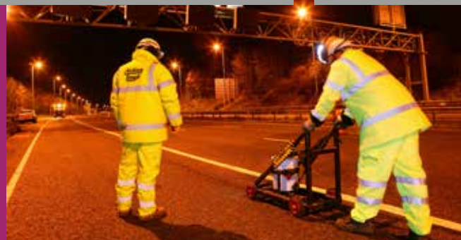
M42 crack infill
