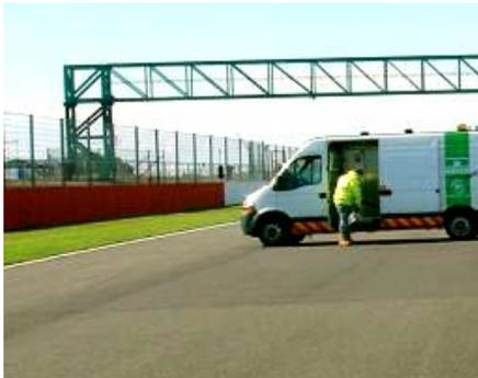
Using one fully-equipped vehicle with a two-man team, Nu-Phalt heated the track wearing course with an infrared emission at the entry level to the previously-repaired section.
