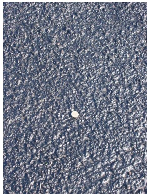
Over a period of time, the action of traffic on the Fortseal System exposes the microtexture of the aggregate restoring it to the original colour and texture, with the Fortseal remaining in the macrotexture of the surface acting as a Preservative and retarding the weathering process.
