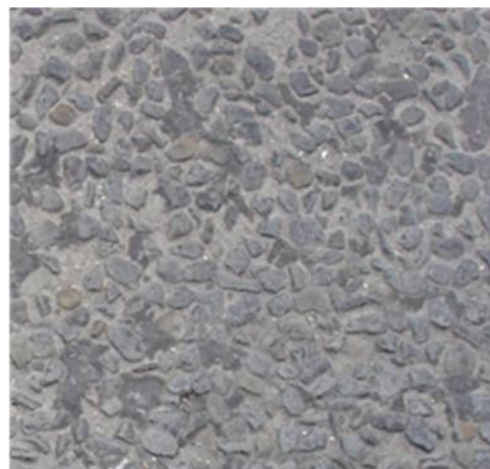
2011 – Showing repair in carriageway after 14 years
