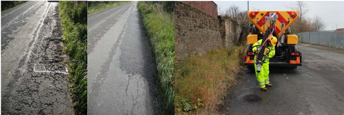
Velocity road repairs are a fast and efficient way to improve the network as the process does not cause any further damage to the road base and the simple but effective solution cleans, seals and repairs road damage extending the life of the carriageway and preventing the main cause of carriageway failure – water from penetrating damaged carriageway.
