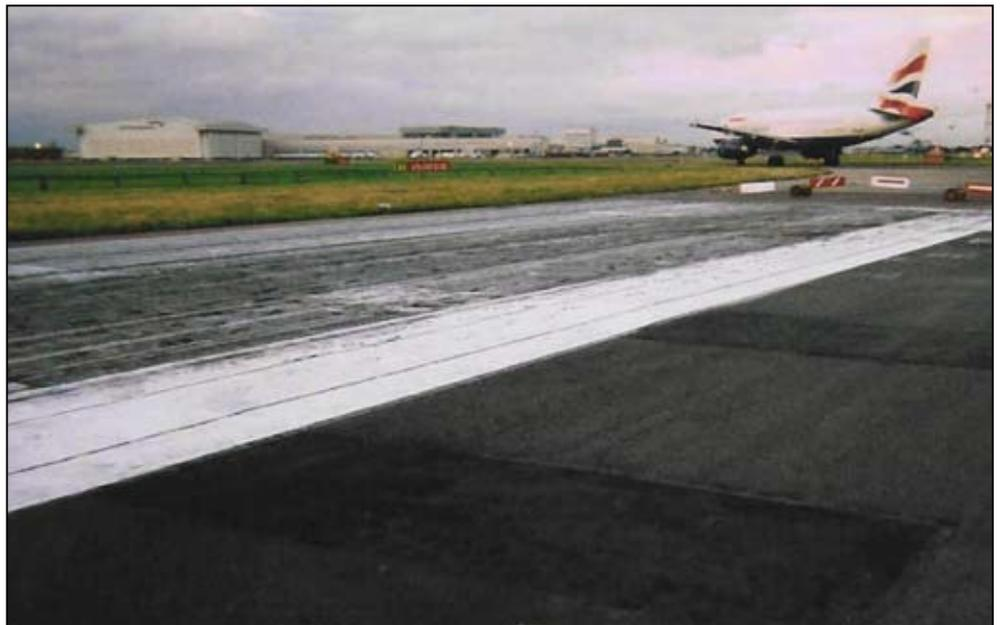
During installation, the textile absorbs bitumen, creating a permanent waterproof barrier. This prevents deterioration caused by water penetration and chemical attack. The high tensile strength, low elongation grid provides permanent, high-performance pavement reinforcement to protect the new overlay against cracking and rutting.
