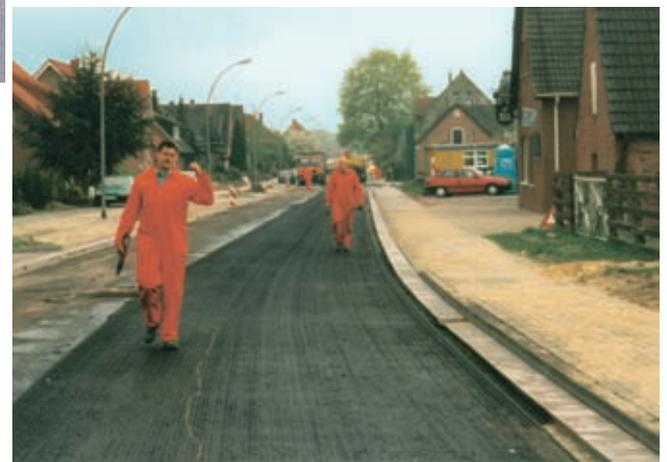
During the works **HaTelit®** was laid in accordance with the **HaTelit®** installation instructions and then covered with 5 cm asphalt-concrete 0/11 surface course.
