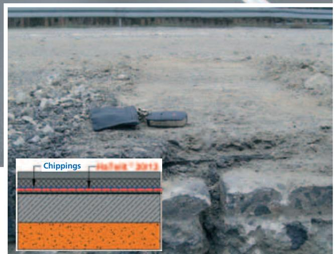
Part of German Highway 13 broken out during reconstruction in 2005 – remaining asphalt binder course above **HaTelit®** – no visible cracks
