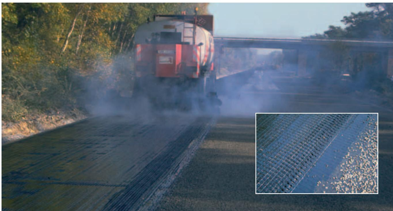
Work in 1990 showing the SAMI being sprayed on to the **HaTelit®** reinforcement grid before chips were spread.
